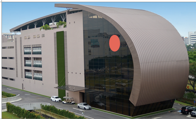
Industrial Building, Singapore
