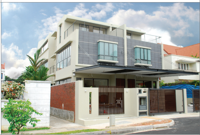
Private House @ Mackerrow Road
