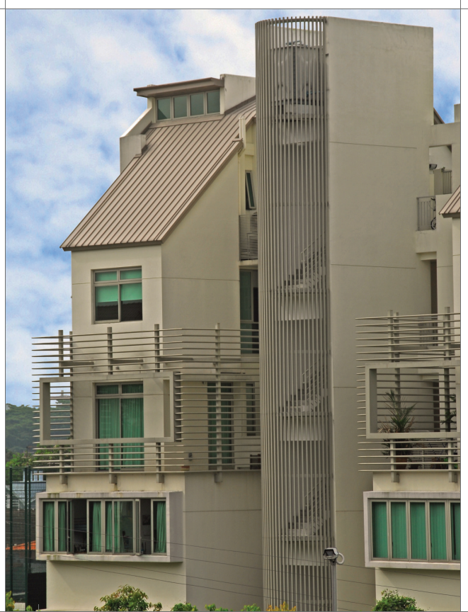
Glentrees Condominium, Singapore
