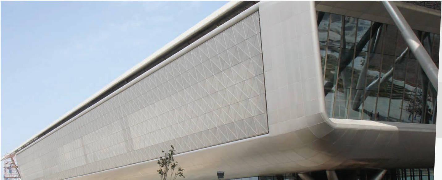
Qatar Foundations Education City - Steel Facade Construction
