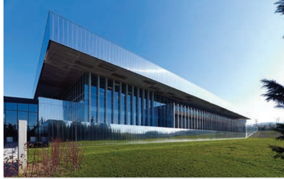
Yapı Kredi Banking Base Mirror Finished Stainless Steel Facade & Expanded Mesh Ceiling
