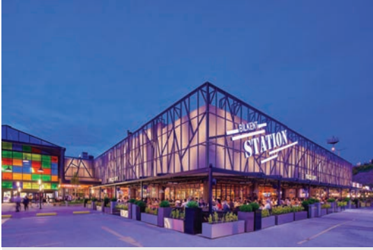
Bilkent Station Powder Coated Aluminum Expanded Mesh Facade
